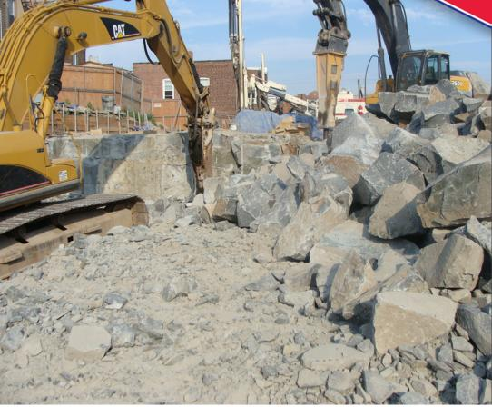
Impact hammers could not break the rock. Da-mite was required to create initial cracks so the hammers could be effective.
