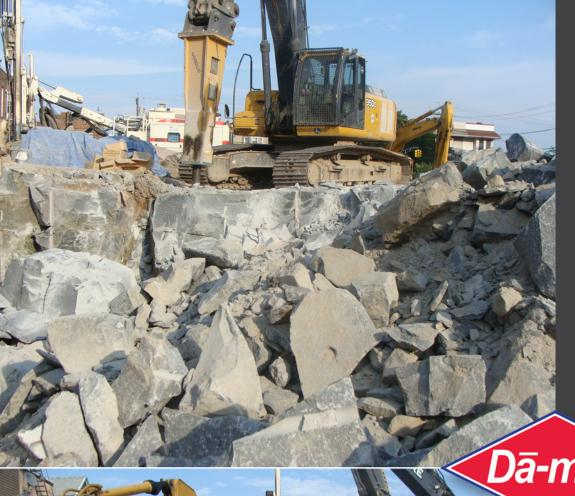
After Da-mite cracked the rock, b/c of the large pieces left, impact hammers were used to further breakdown the rock and separate it from each other.
